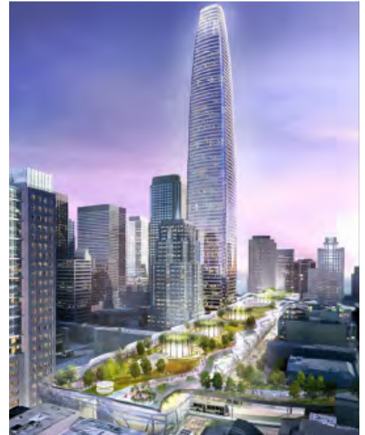
Transbay Terminal in San Francisco, CA.
