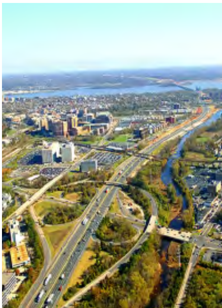
An aerial view of Capital Beltway in Northern VA.
