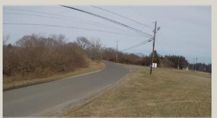
Existing Church Street showing sharp curve with limited sight distance and a lack of pavement markings, signing and shoulders. There is no safe place for pedestrians.
